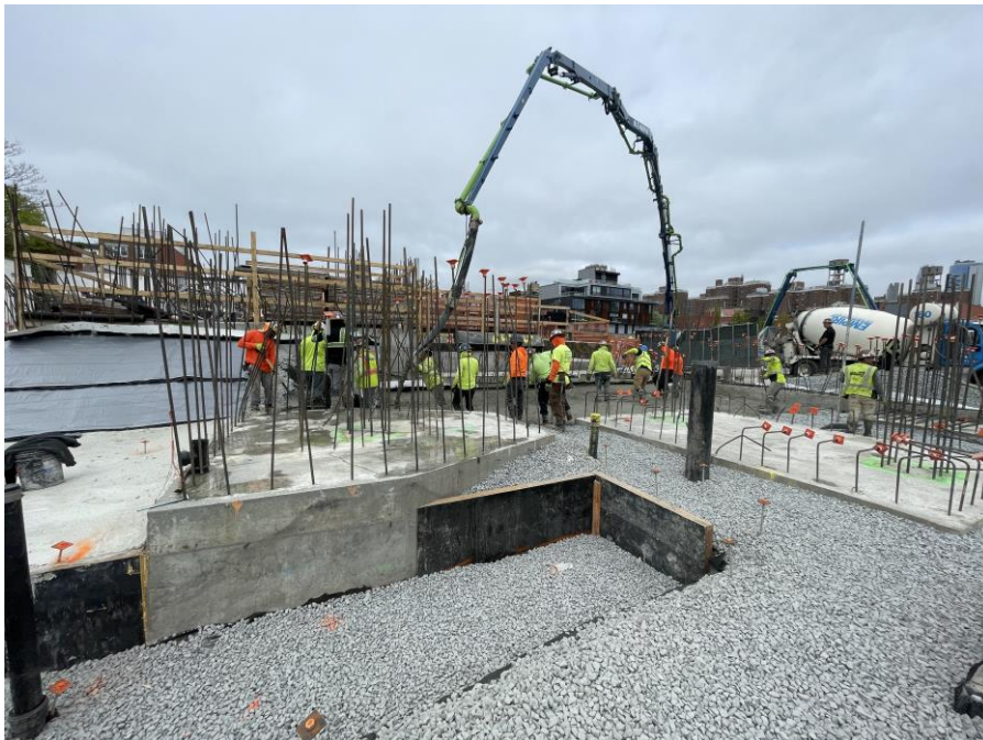
Photo 2: Kingdom placing concrete for a mud slab above the SMD system in the northeastern part of Sackett Place (facing northeast)
