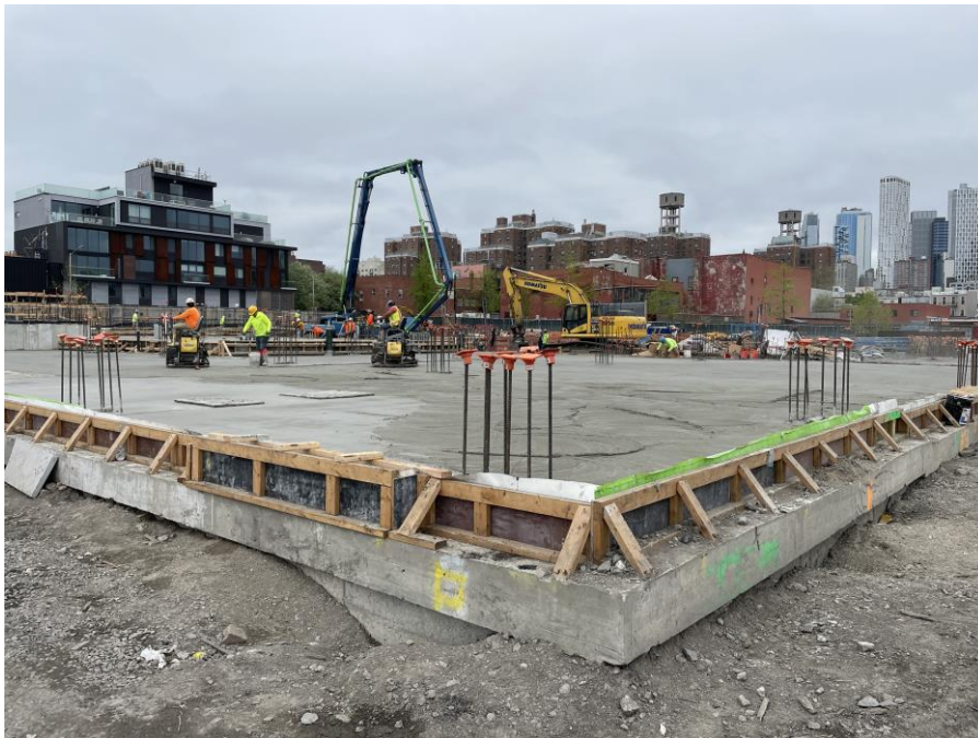
Photo 1: Kingdom placing concrete for the first-floor slab in the northern part of Society Brooklyn (facing north)
