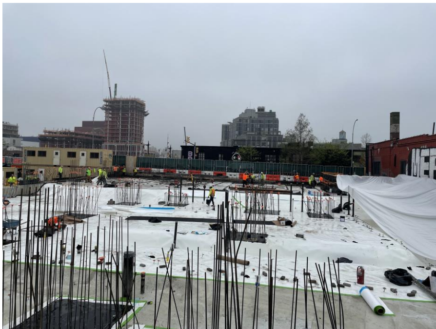
Photo 2: Kingdom installing the waterproofing/vapor barrier membrane in the southern part of Sackett Place (facing south)
