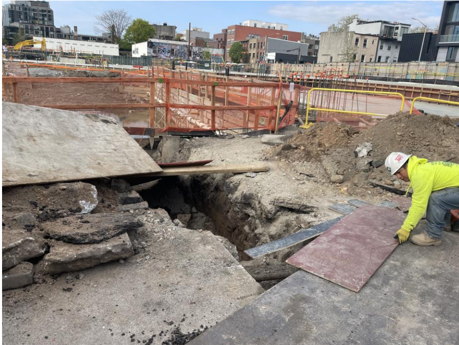
Photo 1: Underground excavating to install utilities in the northern part of Society Brooklyn (facing southwest)
