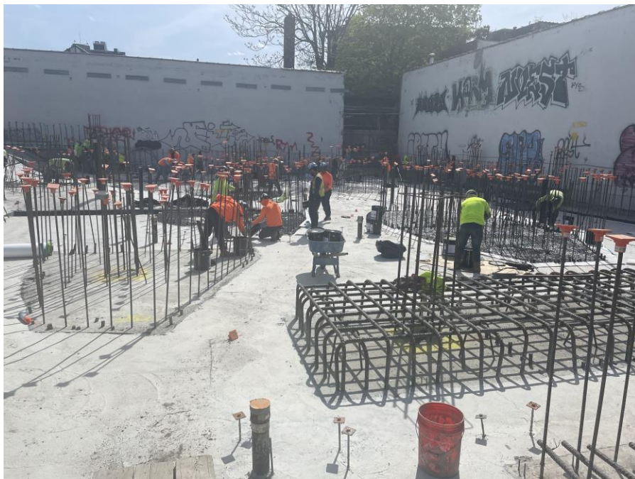
Photo 2: Kingdom installing the waterproofing/vapor barrier membrane in the northeastern part of Sackett Place (facing southwest)
