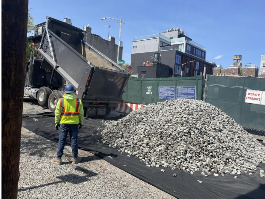
Photo 1: Kingdom placing 2.5-inch virgin quarry stone for the stabilized construction entrance in the northwestern part of Sackett Place (facing north)
