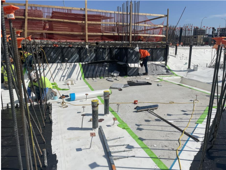
Photo 1: Kingdom installing the waterproofing/vapor barrier membrane in the northern part of Sackett Place (facing northeast)
