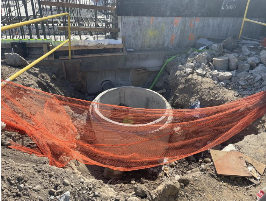
Photo 1: Underground installing utilities within the Sackett Street right-of-way (facing southwest)
