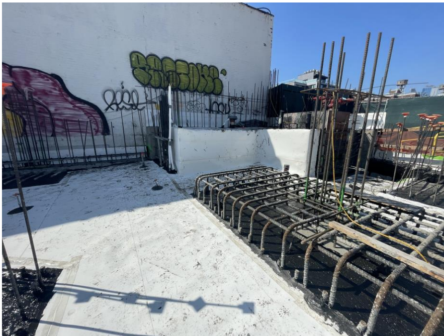
Photo 2: Kingdom installed the waterproofing/vapor barrier membrane in the northwestern part of Sackett Place (facing northwest)
