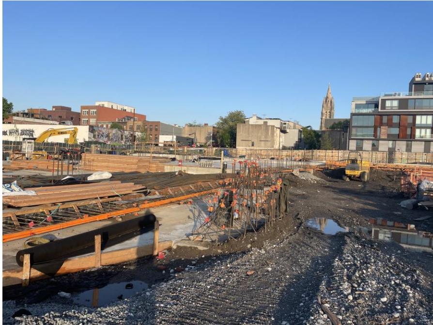
Photo 1: General view of Society Brooklyn (facing southwest)
