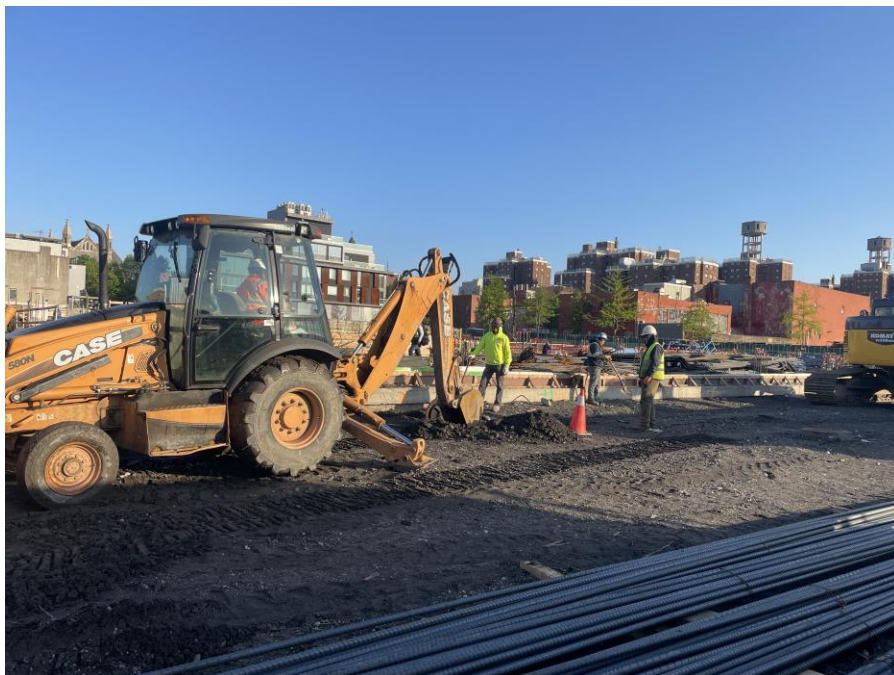
Photo 2: Underground excavating to install utilities in the eastern part of Society Brooklyn within the SPW (facing northwest).
