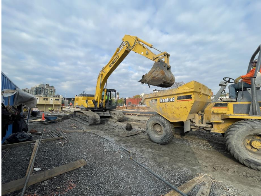
Photo 1: G&M relocating a petroleum-impacted historic fill stockpile in the eastern part of Sackett Place (facing southwest)
