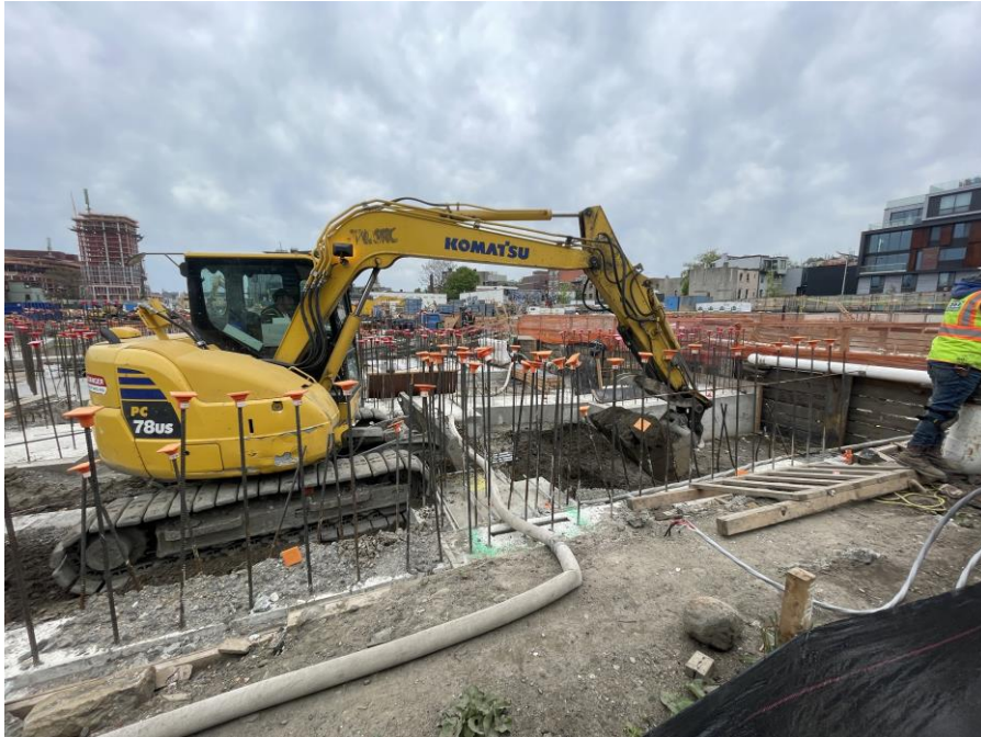
Photo 1: Kingdom excavating to create a level surface for dewatering system equipment in the northern part of Society Brooklyn (facing southwest)
