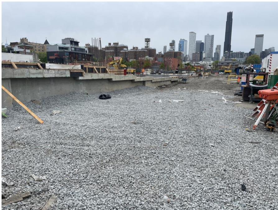
Photo 2: View of ASTM #5 virgin quarry stone backfill in the southern part of Sackett Place within the SPW (facing north)
