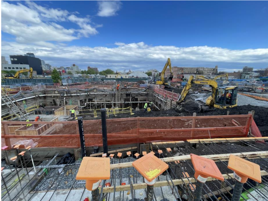
Photo 1: Kingdom excavating for the future cellar in the northern part of Society Brooklyn (facing west)
