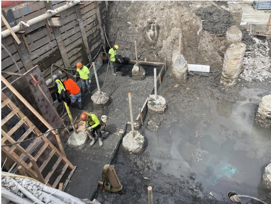
Photo 1: Kingdom applying Petrofix reagent to the base of Remedial Excavation Area No. 1 in the northern part of Society Brooklyn (facing southwest)
