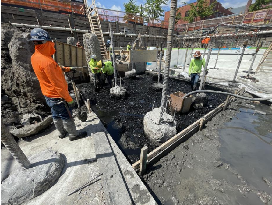
Photo 1: Kingdom applying Petrofix reagent to a portion of the base of Remedial Excavation Area No. 1 in the northern part of Society Brooklyn (facing north)
