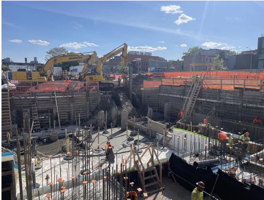
Photo 1: Kingdom excavating for the future cellar in the northern part of Society Brooklyn (facing southwest)
