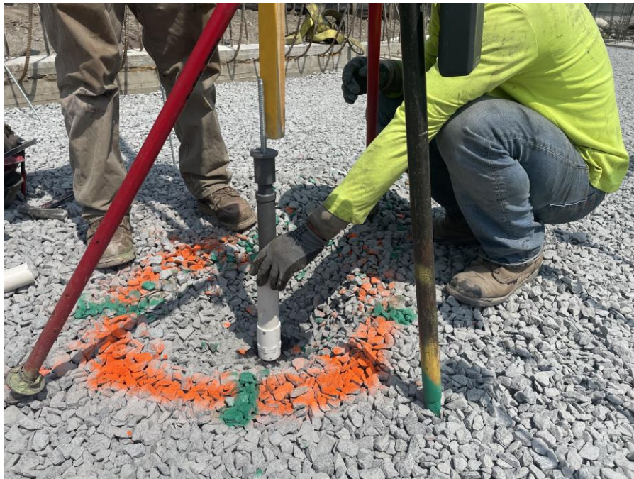
Photo 2: Kingdom installing VMP MP02 in the northeastern part of Society Brooklyn (facing west)
