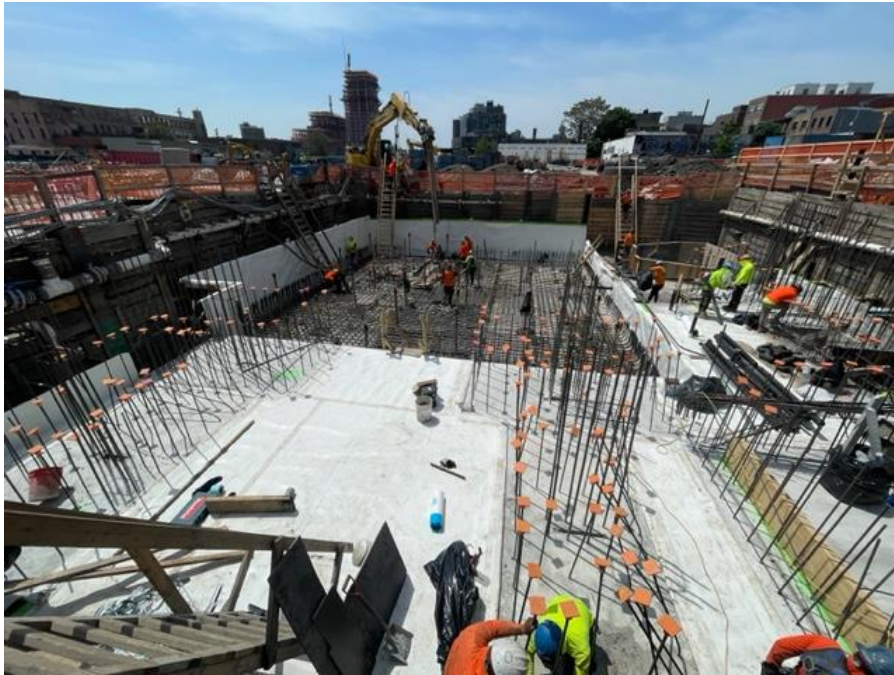
Photo 1: General view of waterproofing progress in the Society Brooklyn northern cellar (facing south)
