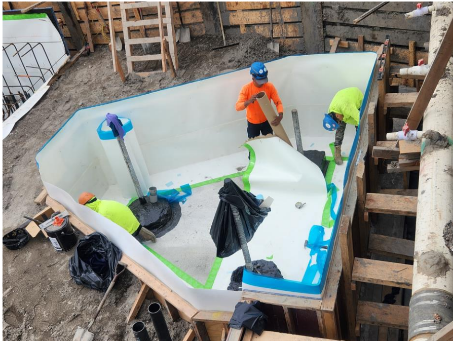
Photo 2: Kingdom installing the waterproofing/vapor barrier membrane in the northern part of Society Brooklyn (facing south)
