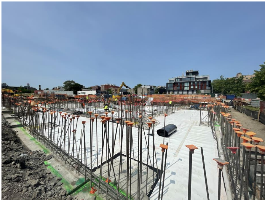
Photo 2: Kingdom installing the waterproofing/vapor barrier membrane in the northern part of Society Brooklyn (facing west)
