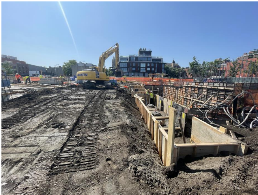
Photo 2: Kingdom grading in the in the northern part of Society Brooklyn (facing west)
