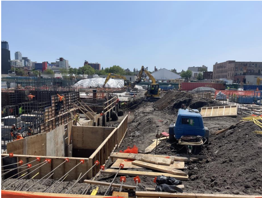
Photo 1: Kingdom excavating to install formwork in the northern part of Society Brooklyn (facing east)
