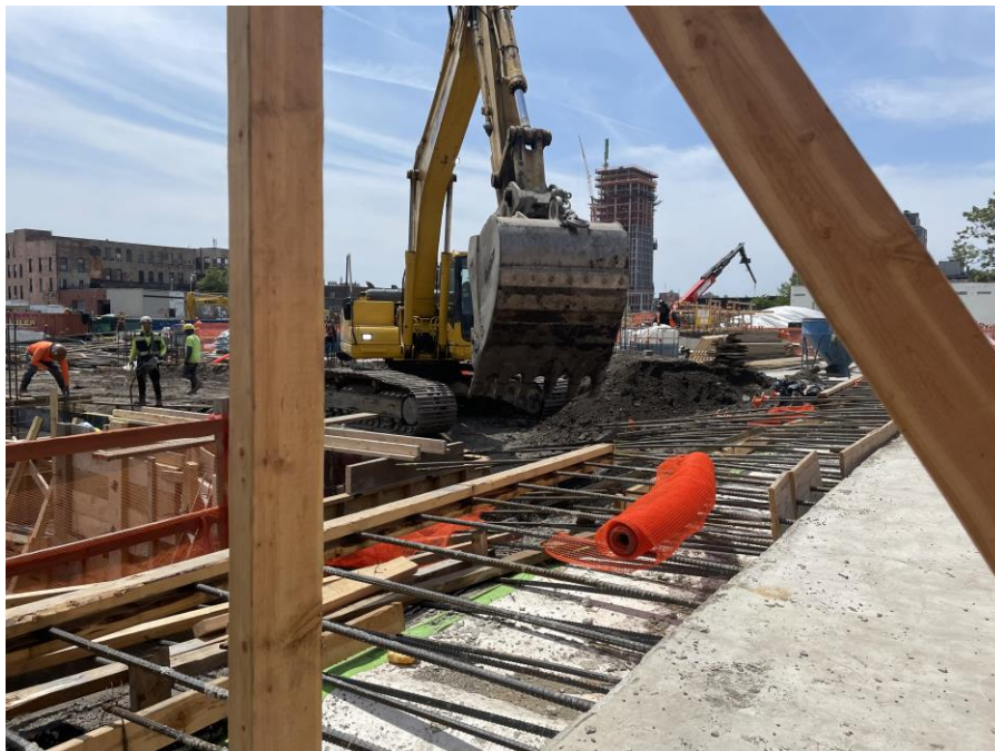
Photo 2: Kingdom backfilling around structural pile cap formwork in the northern part of Society Brooklyn (facing southeast)
