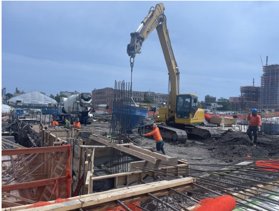
Photo 1: Kingdom placing concrete for structural pile caps in the northern part of Society Brooklyn (facing southeast)
