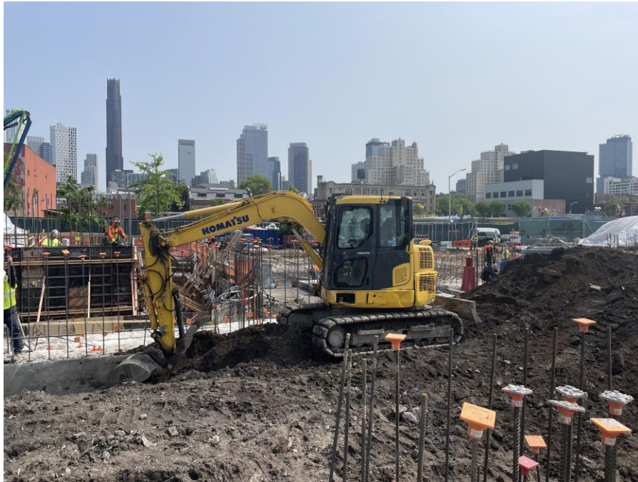
Photo 1: Kingdom excavating to install utilities in the northern part of Society Brooklyn (facing north)
