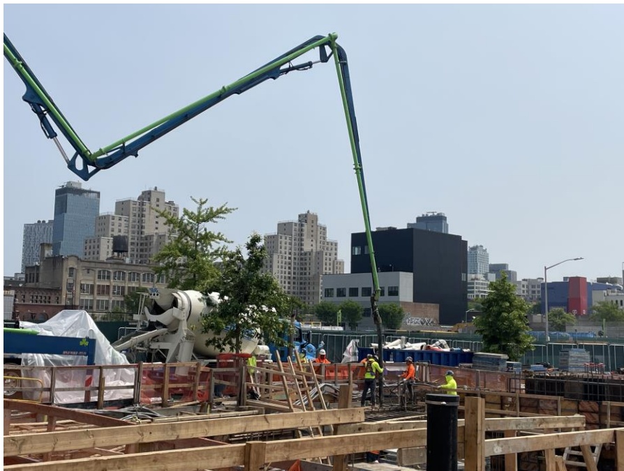
Photo 2: Kingdom placing concrete to install the cellar foundation walls in the northern part of Society Brooklyn (facing north)
