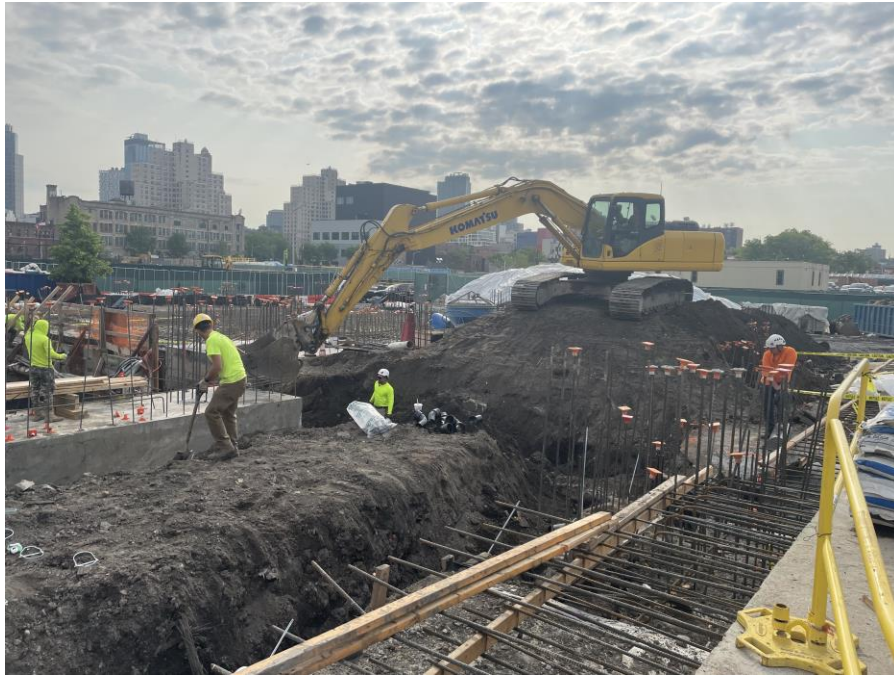
Photo 1: Kingdom excavating to install utilities in the northern part of Society Brooklyn (facing east)
