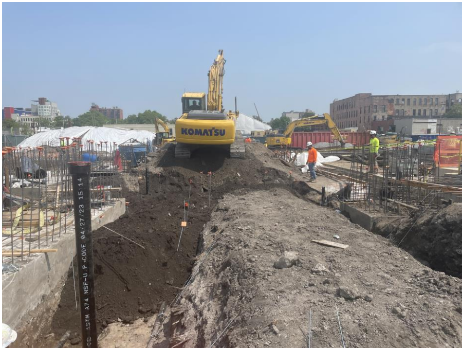
Photo 1: Kingdom backfilling around structural pile caps in the northern part of Society Brooklyn (facing east)
