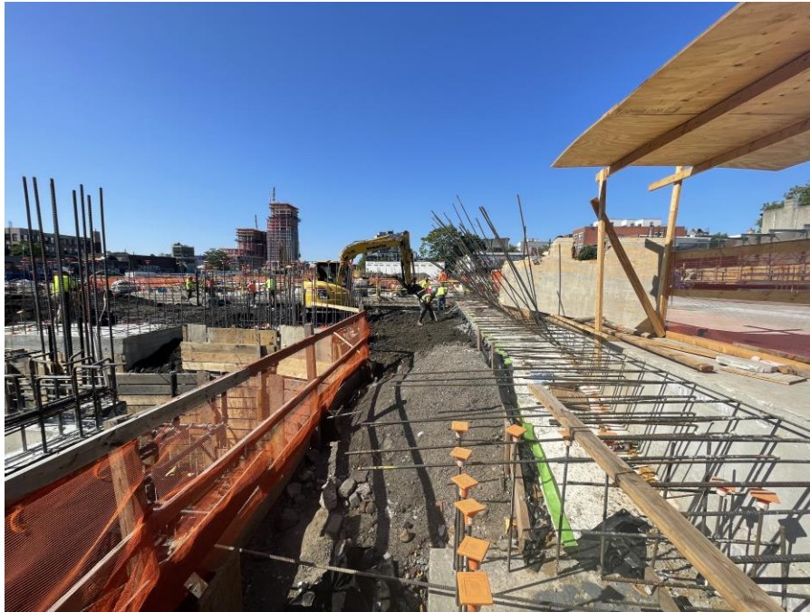
Photo 1: Kingdom backfilling around utilities in the northern part of Society Brooklyn (facing south)
