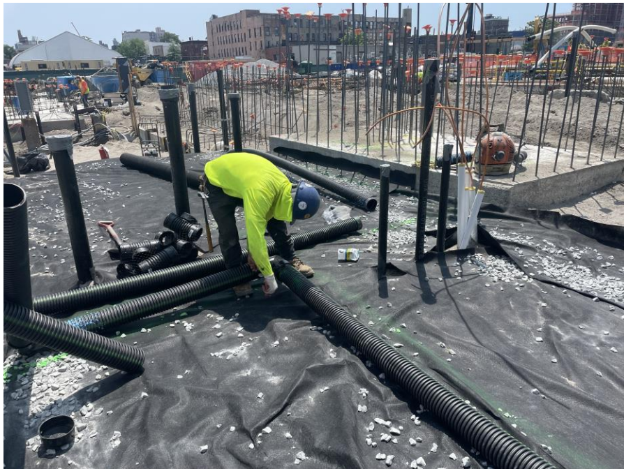
Photo 2: Kingdom installing SMD system components in the northern part of Society Brooklyn (facing southeast)
