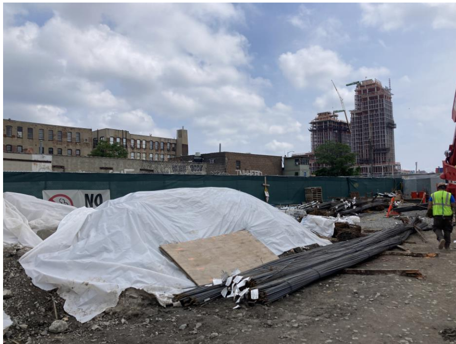
Photo 2: View of stockpile covered with polyethylene sheeting within the SPW (facing southeast)
