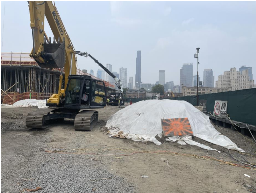
Photo 2: Stockpiled soil covered with polyethylene sheeting within the SPW (facing north)
