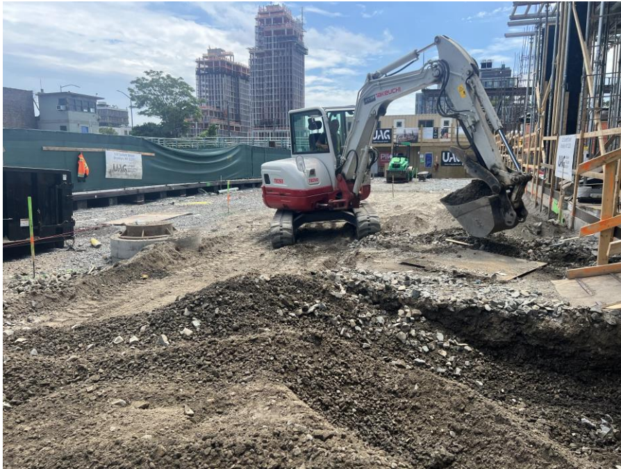
Photo 1: G&M excavating to install the composite cover system in the southeastern part of Sackett Place within the SPW (facing south)
