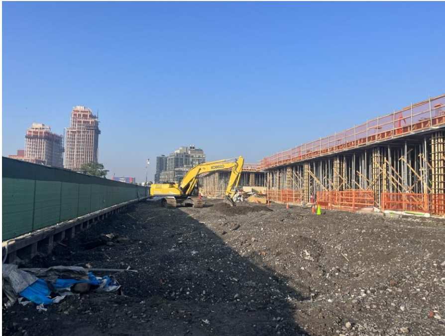
Photo 1: G&M excavating to install the composite cover system in the southeastern part of Society Brooklyn within the SPW (facing southeast)
