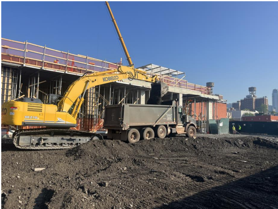
Photo 2: Kingdom exporting non-hazardous soil/fill in permitted tri-axle trucks in the northeastern part of Society Brooklyn within the SPW (facing north)
