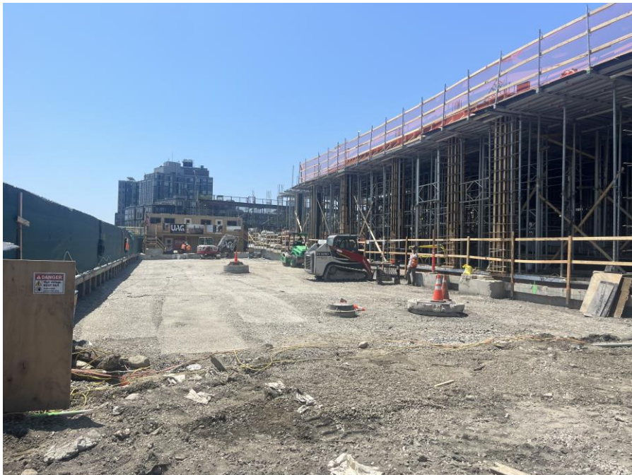
Photo 2: G&M grading to install the temporary composite cover system in the southeastern part of Sackett Place within the SPW (facing south)
