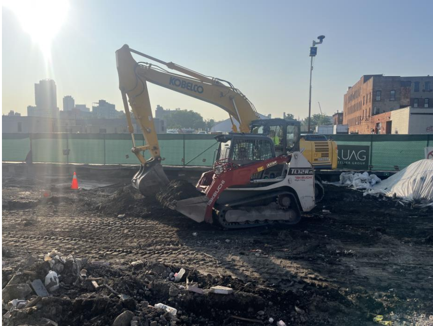
Photo 1: G&M excavating to install the temporary composite cover system in the northeastern part of Sackett Place within the SPW (facing east)
