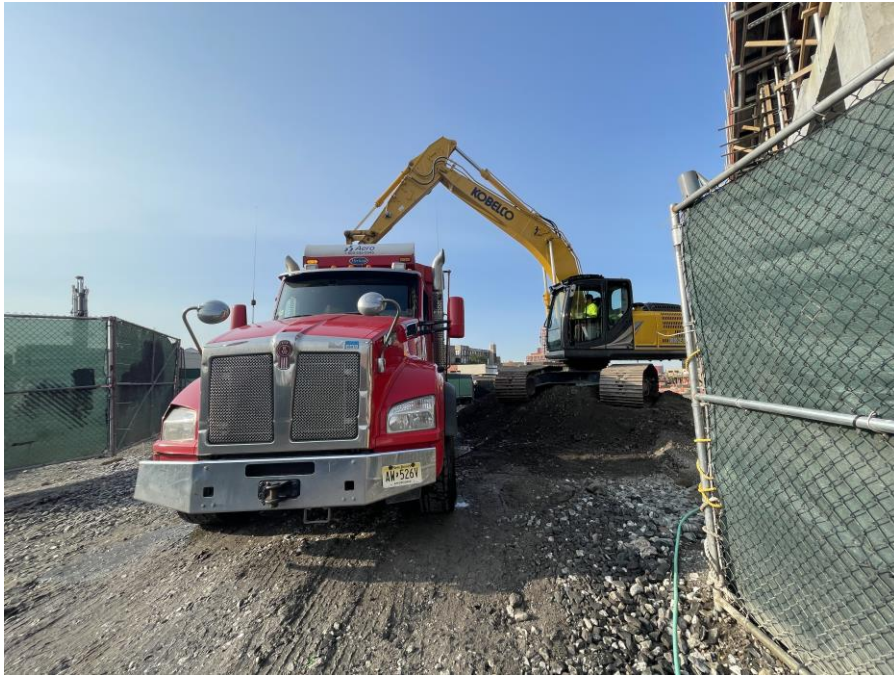
Photo 1: G&M exporting non-hazardous soil/fill in permitted tri-axle trucks in the northeastern part of Society Brooklyn within the SPW (facing south)
