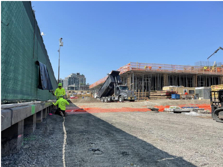
Photo 2: G&M importing 0.5-inch crushed stone for the temporary composite cover system in the southeastern part of Sackett Place within the SPW (facing southwest)
