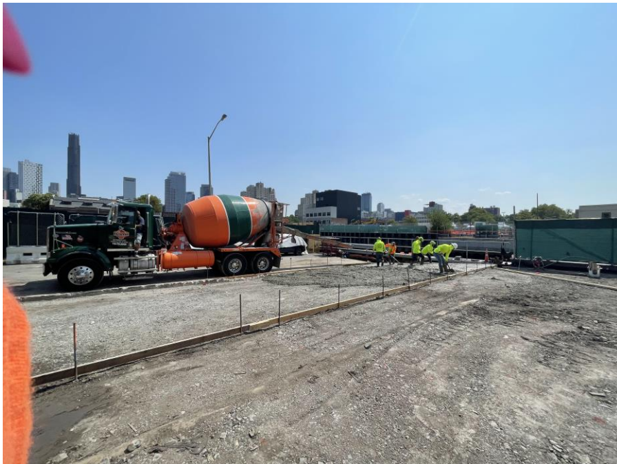
Photo 2: G&M placing concrete for the temporary composite cover system in the northeastern part of Society Brooklyn within the SPW (facing southwest)
