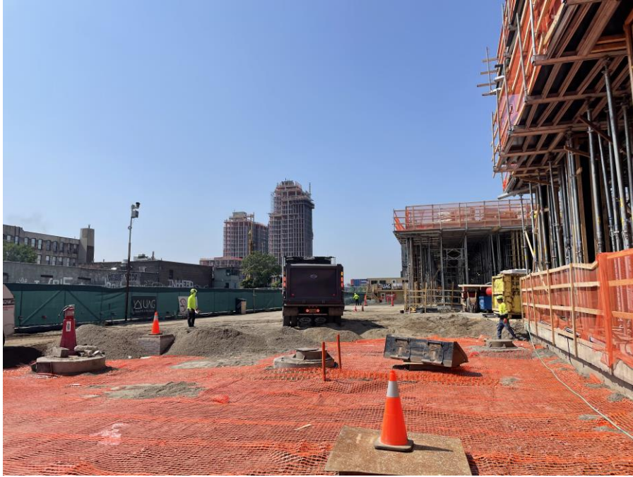
Photo 1: G&M importing 0.5-inch crushed stone for the temporary composite cover system in the southeastern part of Society Brooklyn within the SPW (facing south)
