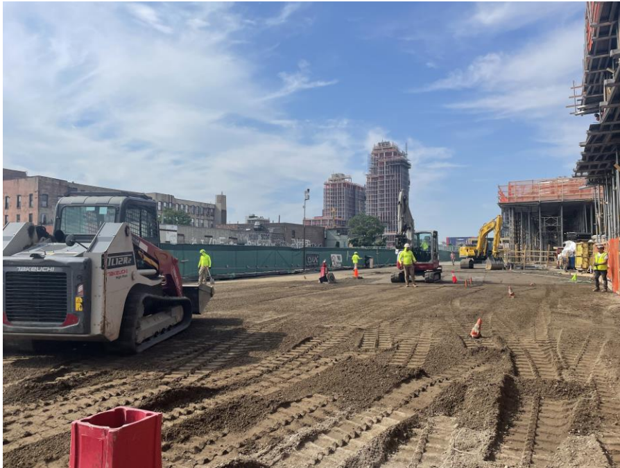
Photo 1: G&M backfilling with 0.5 crushed stone for the temporary composite cover system in the southeastern part of Society Brooklyn within the SPW (facing south)
