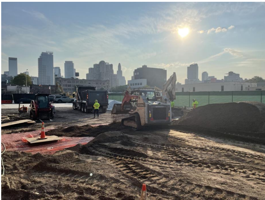
Photo 2: G&M importing 0.5-inch crushed stone for the temporary composite cover system in the eastern part of Society Brooklyn within the SPW (facing northeast)
