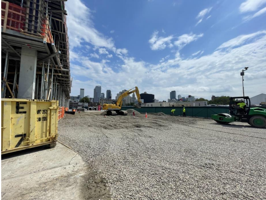
Photo 1: G&M placing 0.75-inch crushed stone for the temporary composite cover system in the eastern part of Society Brooklyn within the SPW (facing northeast)
