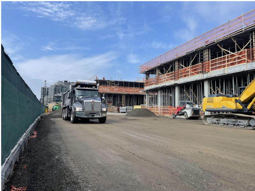
Photo 2: G&M importing 0.75-inch crushed stone for the temporary composite cover system in the eastern part of Society Brooklyn within the SPW (facing southwest)
