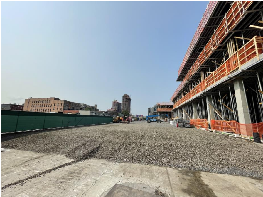
Photo 2: View of the temporary composite cover system in the northeastern part of Society Brooklyn within the SPW (facing south)
