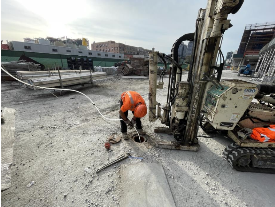
Photo 1: AARCO developing recovery well RW01 in the northeastern part of Society Brooklyn within the shore public walkway (SPW) (facing southeast)
