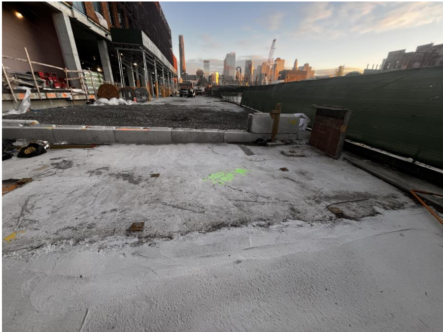
Photo 2: General view of the SPW (facing northeast)
