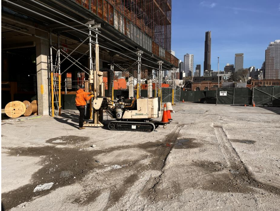
Photo 1: Lakewood advancing soil boring SPW_WC05C in the northeastern part of Society Brooklyn within the SPW (facing north)
