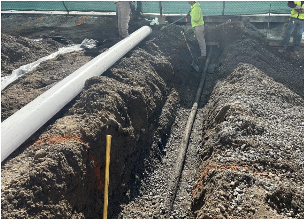
Photo 2: G&M excavated to expose a tie rod in the southern part of Sackett Place within the SPW (facing east)
