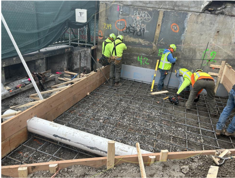
Photo 1: G&M installing formwork in the southern part of Sackett Place within the SPW (facing south)
