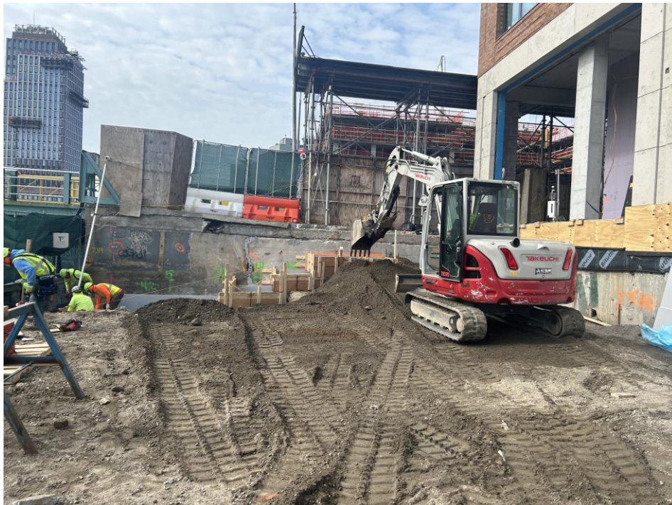
Photo 2: G&M backfilling with previously imported NYSDEC-approved fill and non-impacted historic fill around concrete formwork in the southern part of Sackett Place within the SPW (facing southeast)
