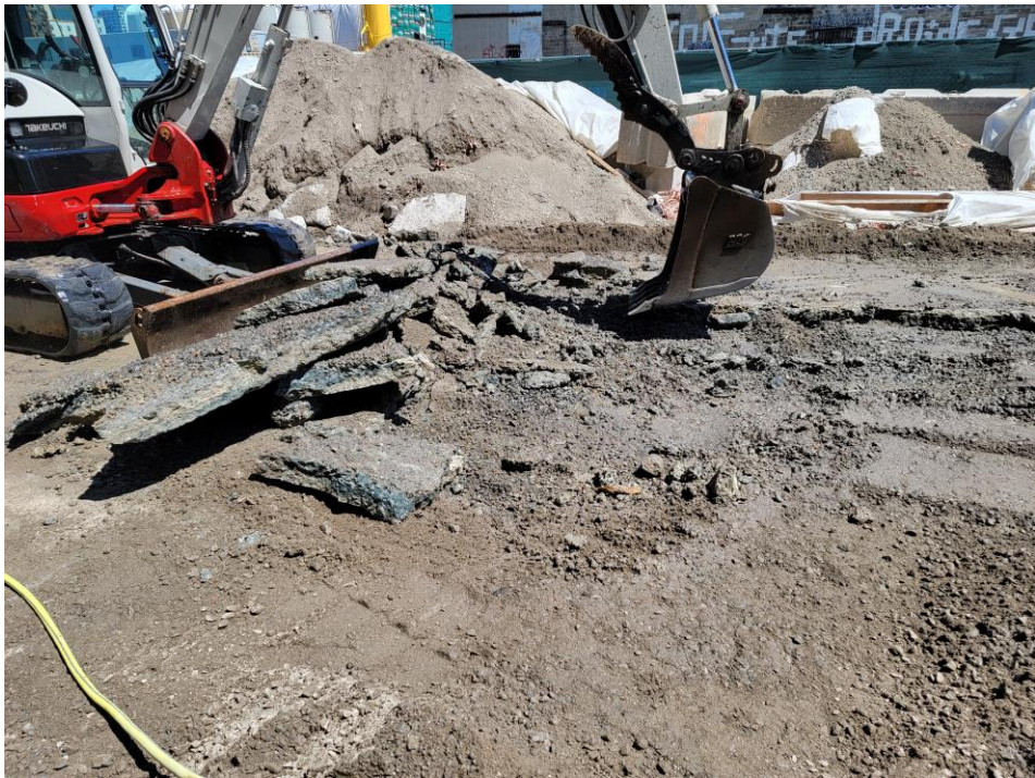
Photo 2: G&M demolishing concrete slab in the eastern part of Sackett Place within the SPW (facing east)
