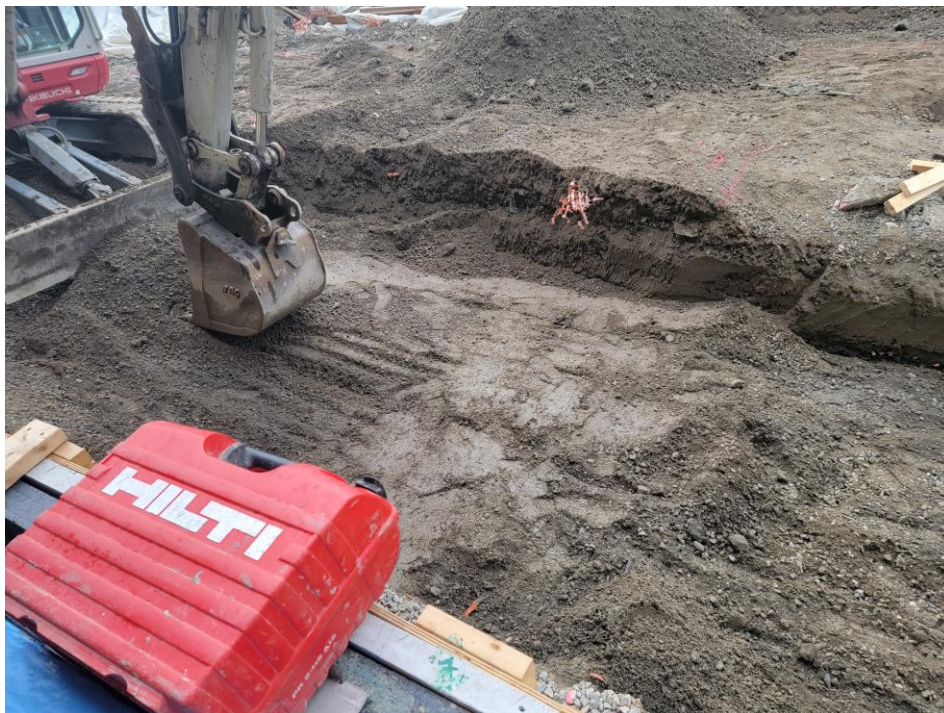
Photo 2: G&M excavating to install foundation elements in the eastern part of Sackett Place within the SPW (facing northeast)
