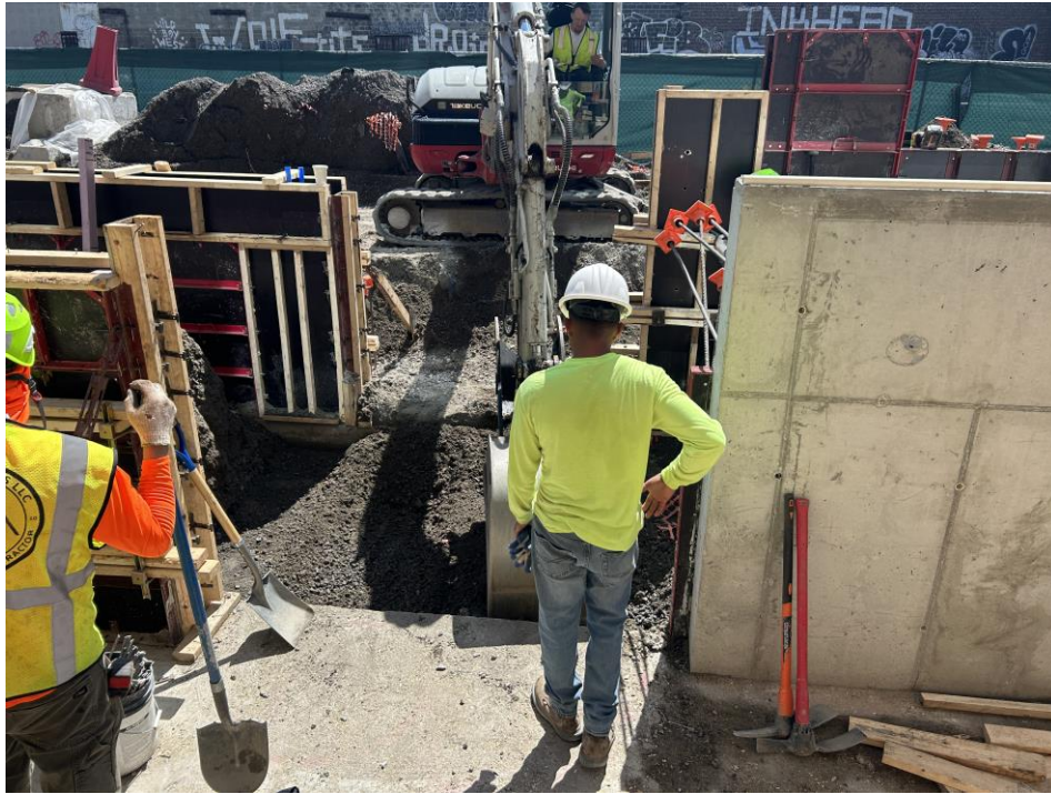
Photo 1: G&M excavating to install foundation elements in the eastern part of Sackett Place within the SPW (facing east)
