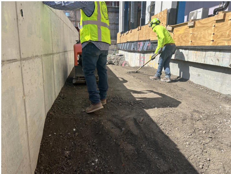
Photo 2: G&M compacting area backfilled with NYSDEC-approved fill and historic fill in the southern part of Sackett Place within the SPW (facing south)
