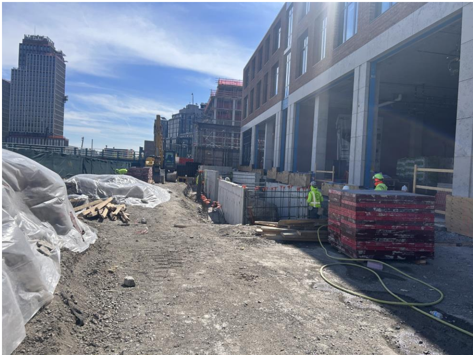
Photo 1: General view of work area (facing south)
