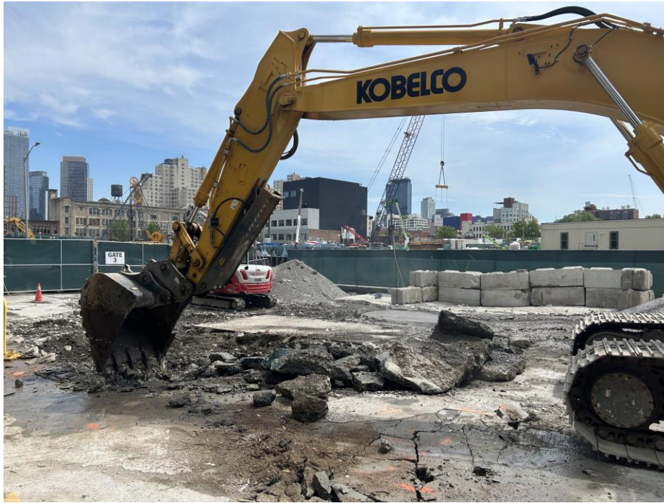
Photo 1: G&M demolishing a concrete slab in the northeastern part of Society Brooklyn within the SPW (facing northeast)
