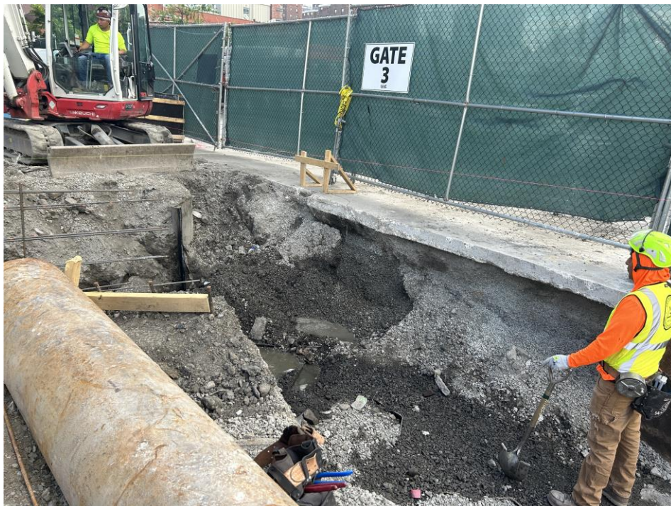
Photo 2: G&M excavating to install foundation elements in the northeastern part of Society Brooklyn within the SPW (facing north)
