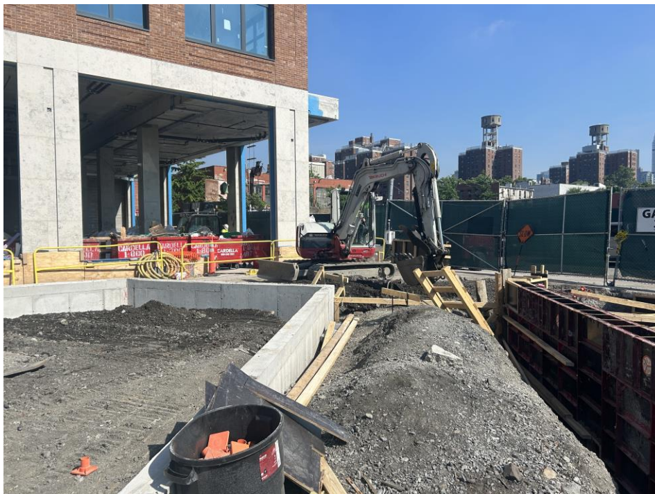
Photo 2: G&M grading to install foundation elements in the northeastern part of Society Brooklyn within the SPW (facing north)
