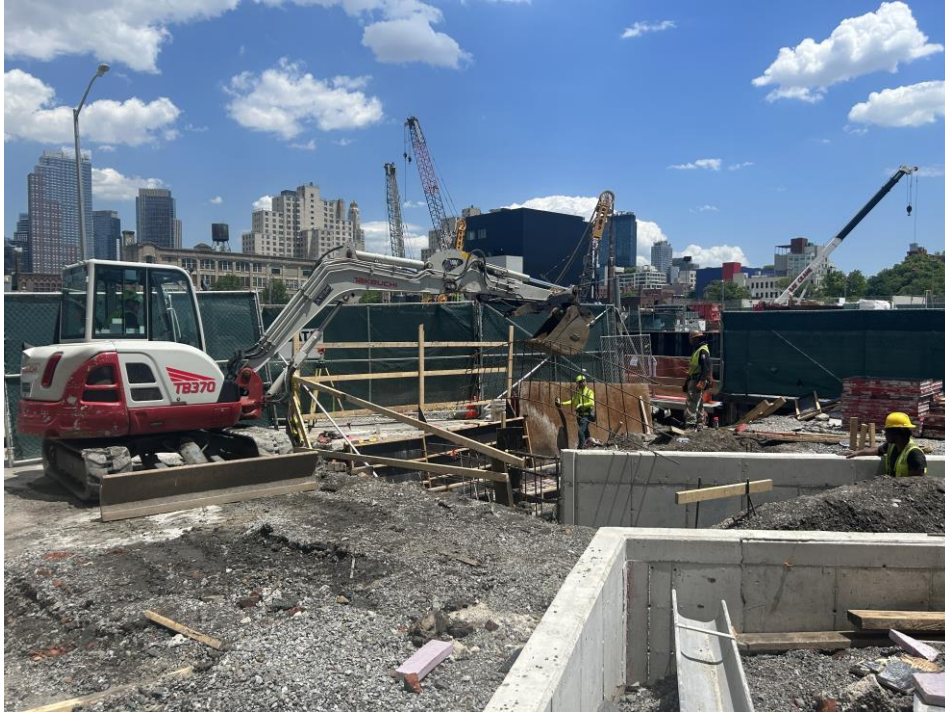
Photo 1: General view of the work area (facing northeast)
