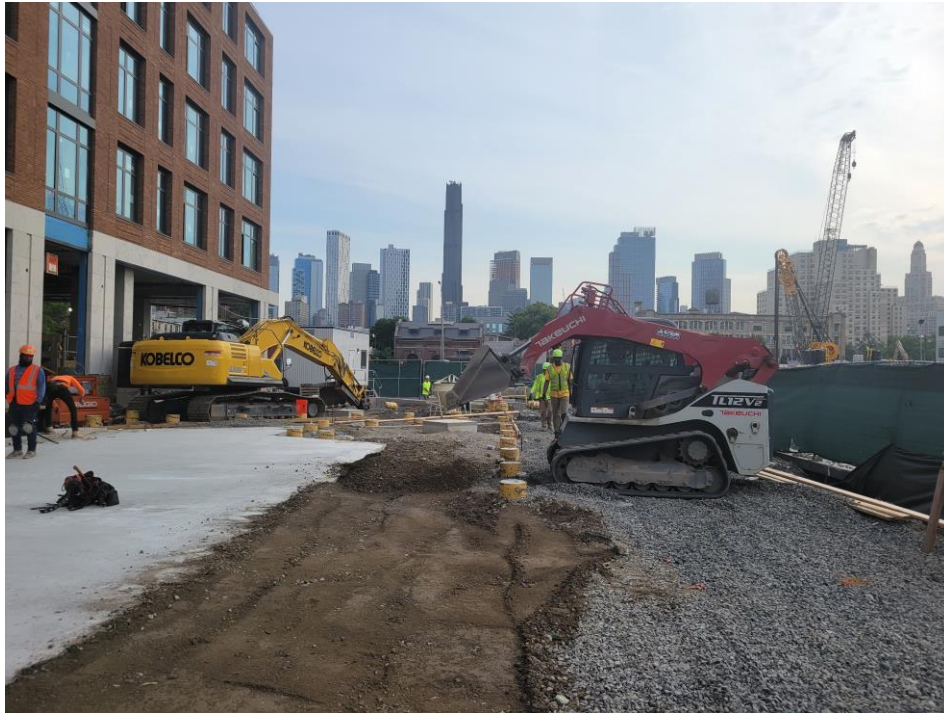
Photo 1: G&M grading in the northeastern part of Society Brooklyn within the SPW (facing north)
