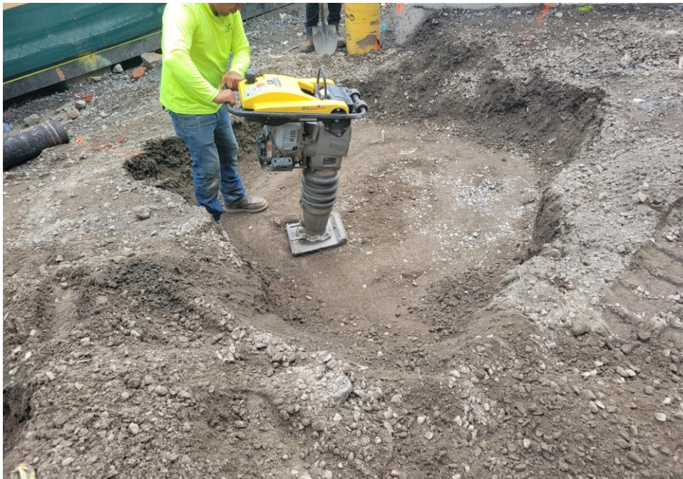
Photo 2: G&M backfilling and compacting in the southeastern part of Sackett Place within the SPW (facing southeast)
