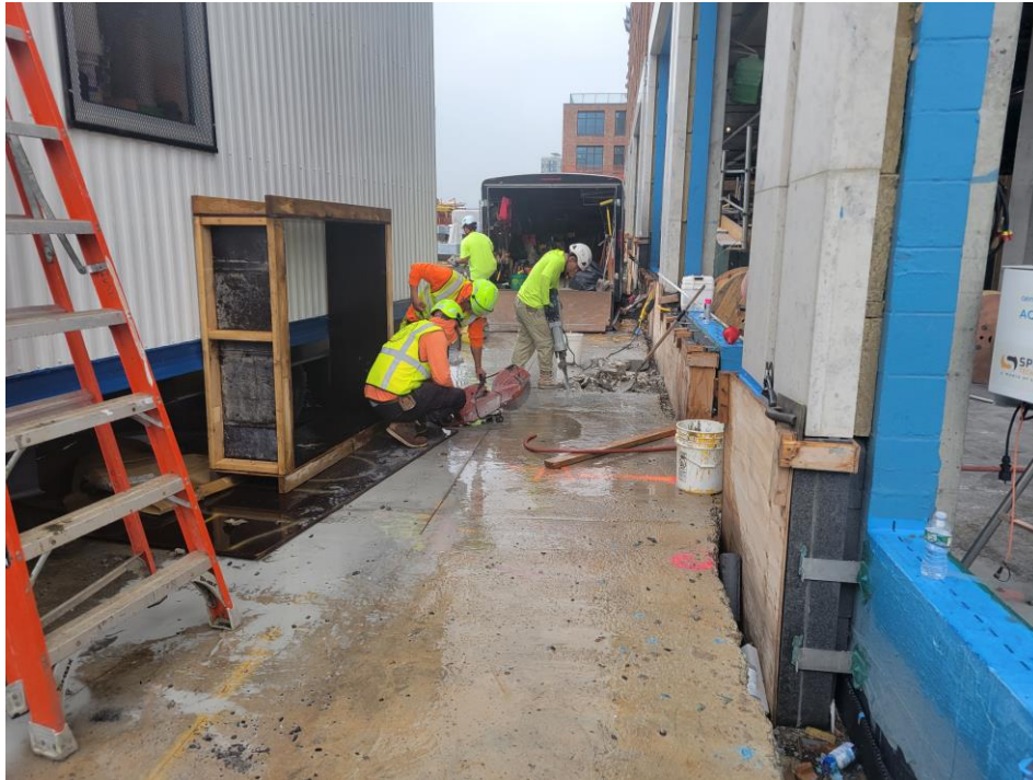
Photo 1: G&M removing a concrete slab in the northeastern part of Society Brooklyn within the SPW (facing south)
