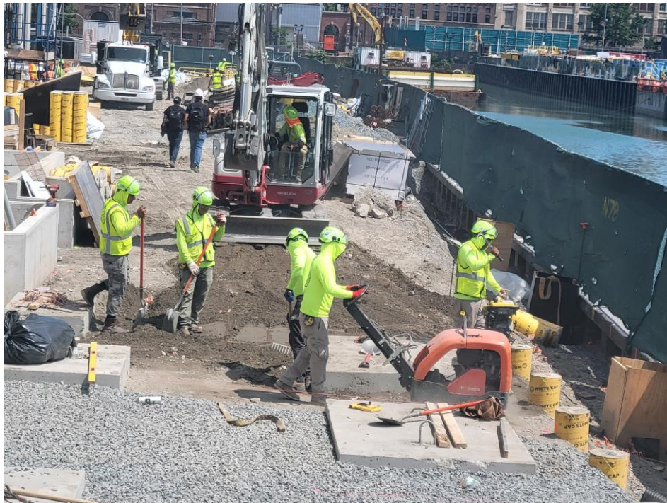
Photo 2: G&M backfilling with NYSDEC-approved fill in the southeastern part of Sackett Place within the SPW (facing north)
