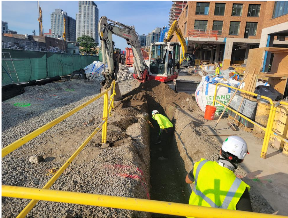
Photo 1: G&M excavating for utility installation in the northeastern part of Society Brooklyn within the SPW (facing south)
